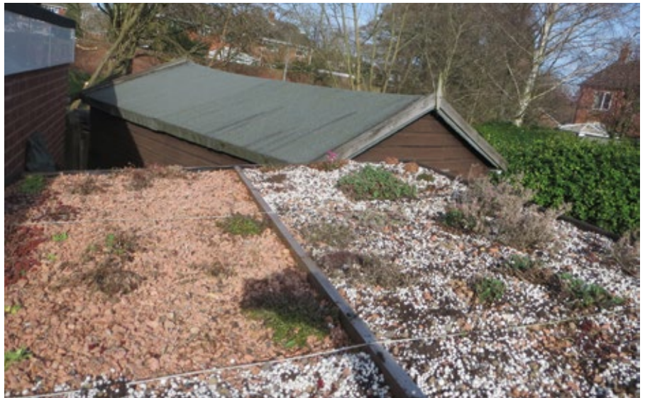
Fig 9: The roof mid-way through the spring renovations
