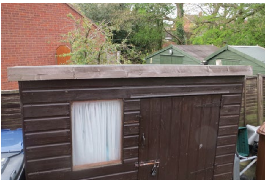
Fig 2: The shed used for the green roof
