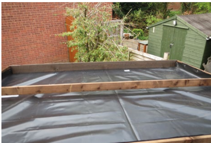
Fig 4: PVC liner added to roof and tacked in place
