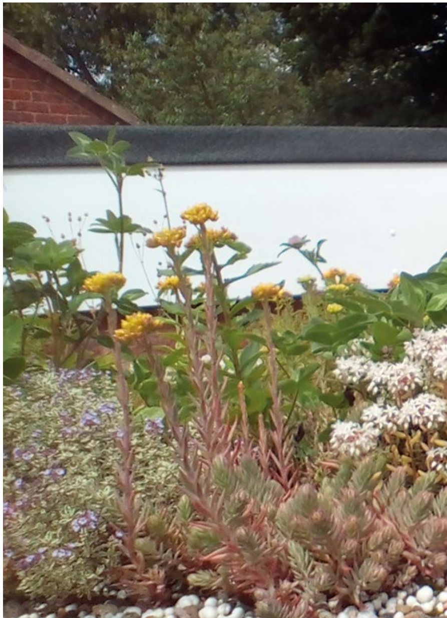
Fig 10: Green roof in summer 2016
