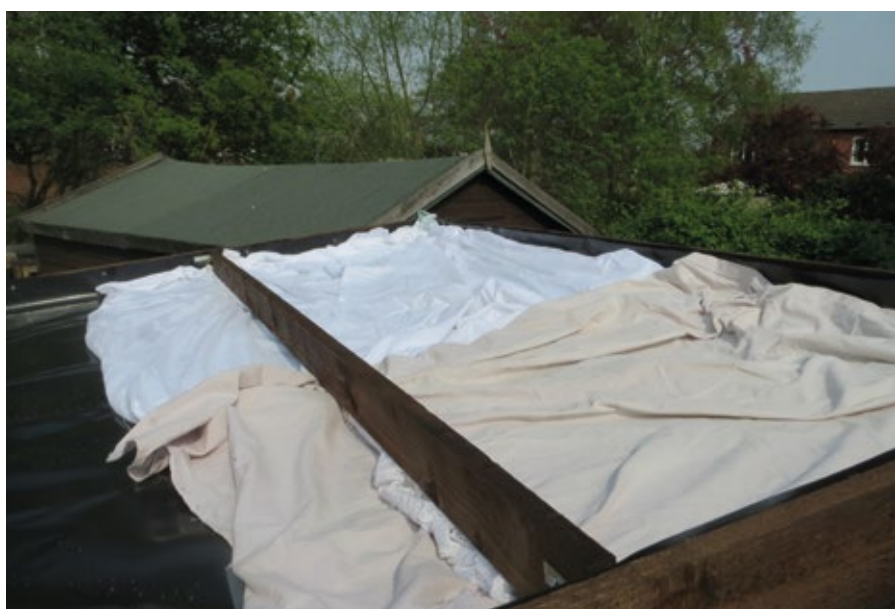
Fig 5: Old sheets used to protect PVC liner
