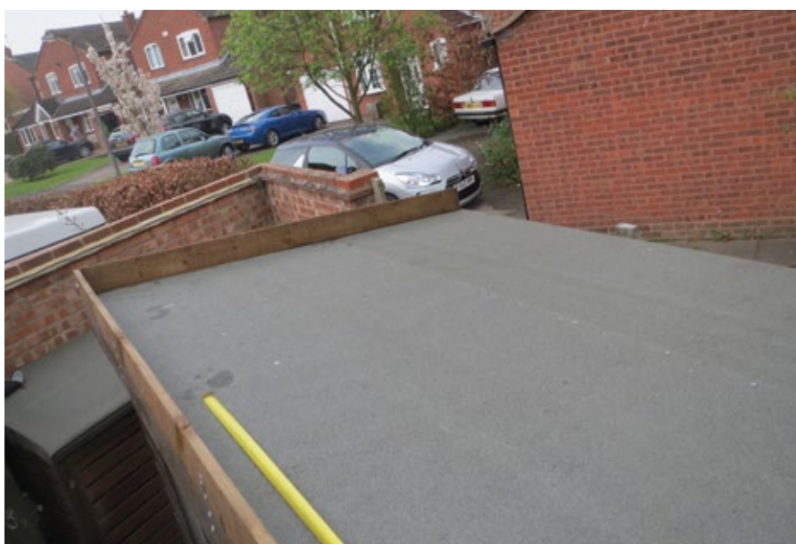
Fig 3: Wooden box constructed on existing roof
