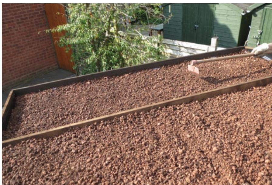
Fig 6: Substrate added to roof and raked in
