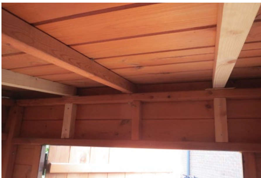
Fig 1: Wooden battens used as additional support for roof
